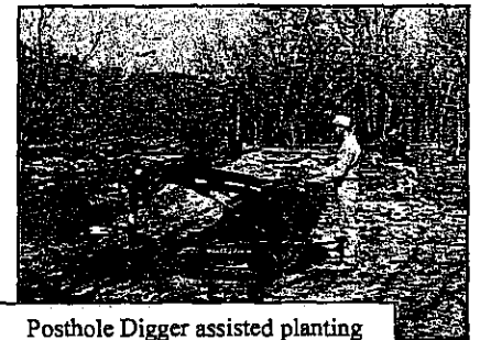
Posthole Digger assisted planting 10-gallon trees & shrubs.
